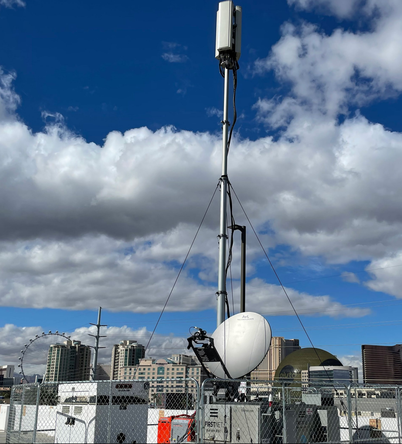
The FirstNet Authority's pre-planning program helps public safety identify areas they may need coverage augmentation during large planned events, such as this Satellite Cell on Light Truck put on hot standby during Super Bowl LVIII in Las Vegas.
